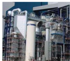
WTA® Lignite pre drying process
